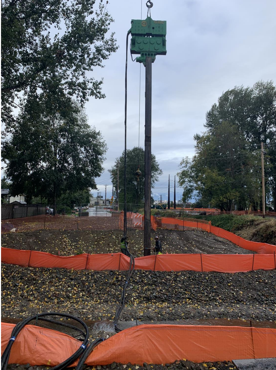
Bridge piling installation.
