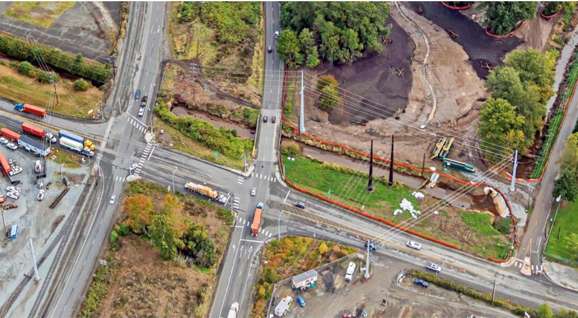
Power Pole structures 1, 2 & 3 in place with lines strung.
